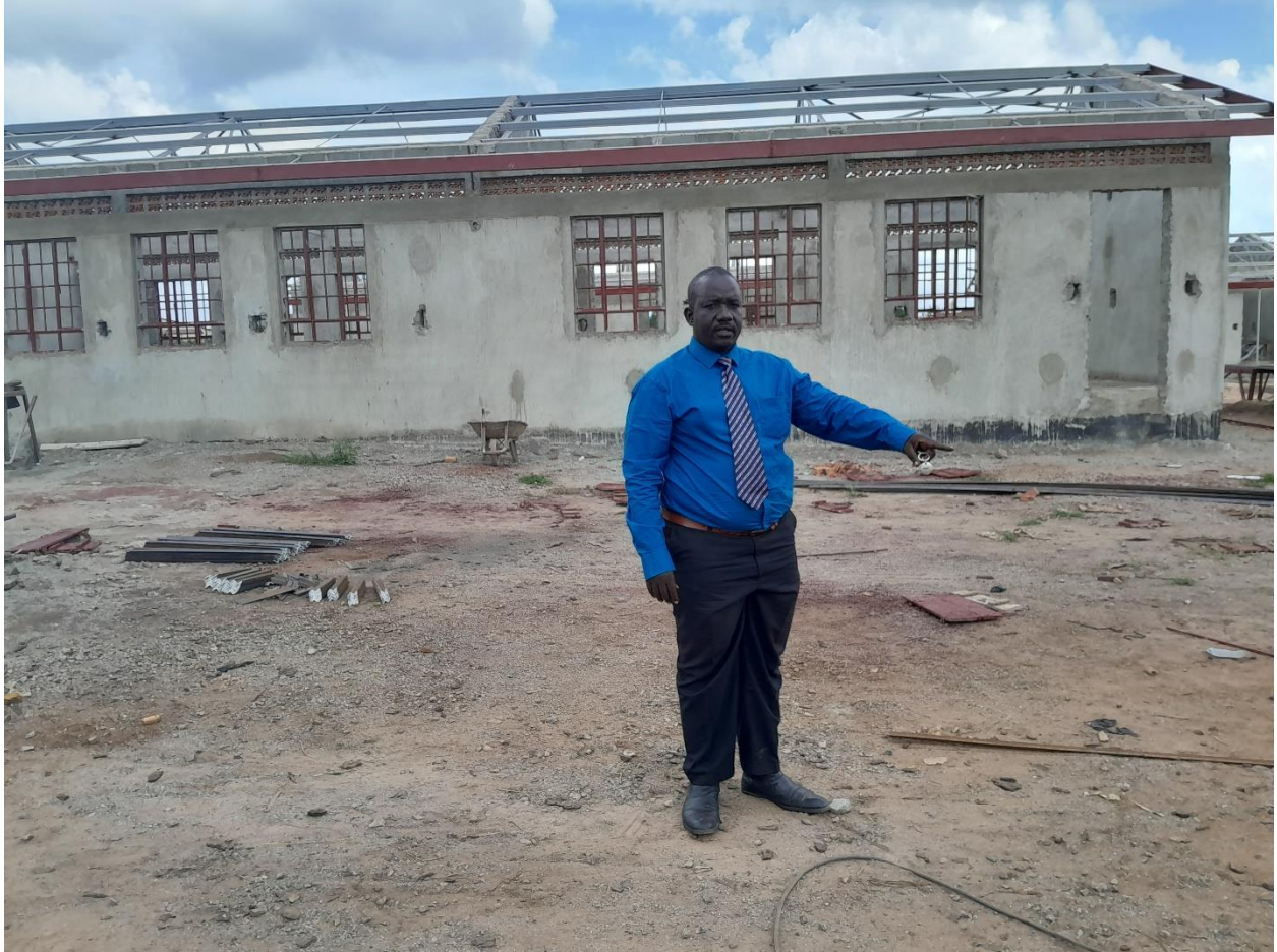
Monitoring construction works at Railway Seed secondary school
