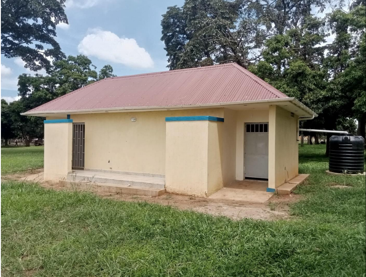
Stance Drainable latrine with the section for PWD
