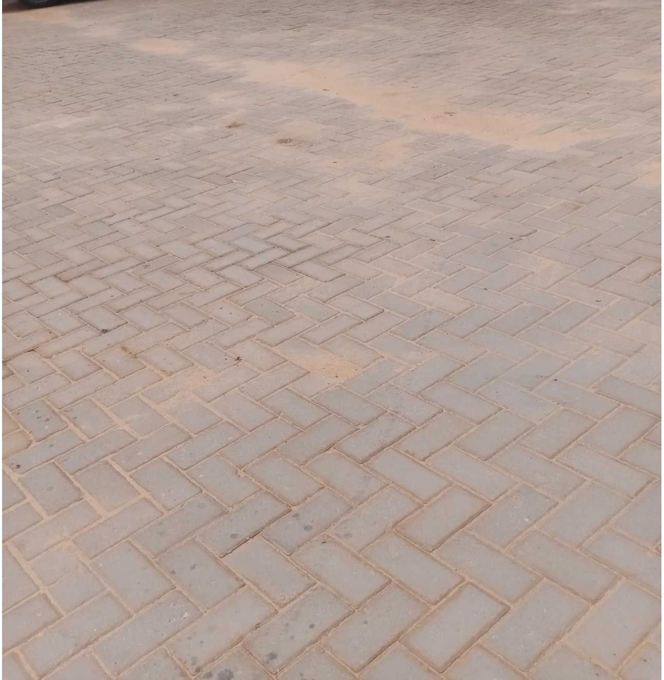
Pavers at the compound of Lira city Council
