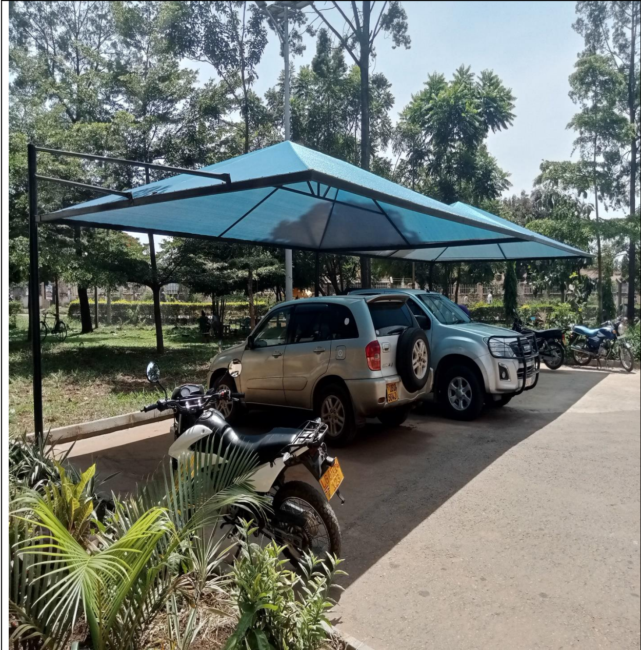
The erected Vehicle Shed Canopy
