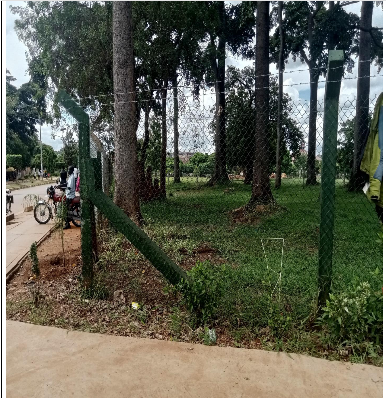
Erected Chain-Link Using Chain Block Machine
