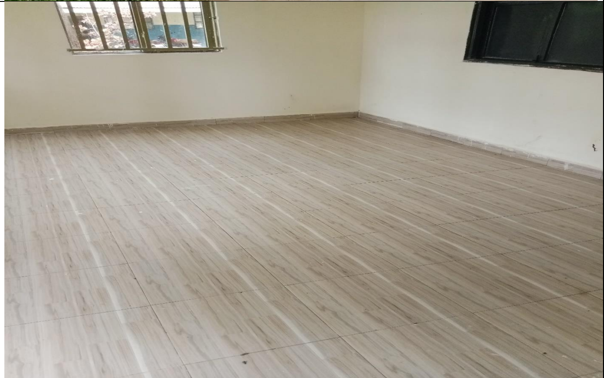
Canteen and the Interior Tiling
